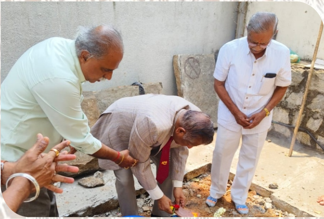
Digging Borewell @ APS Premisis
