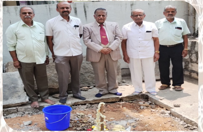
Digging Borewell @ APS Premisis
